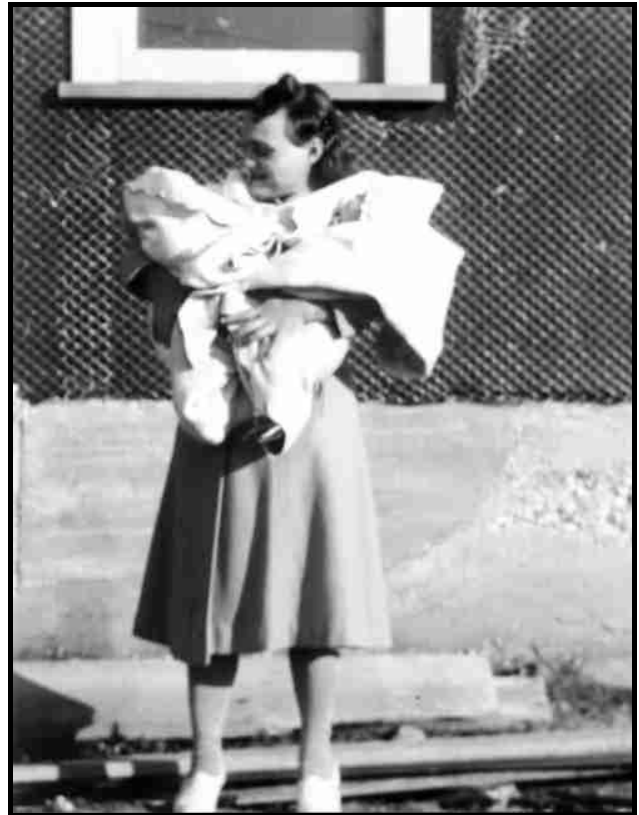
Norma Woodruff holding the twins. Notice the boards and walls of the new house. While the family lived in the basement, Richard built a house overhead. - Summer 1941
